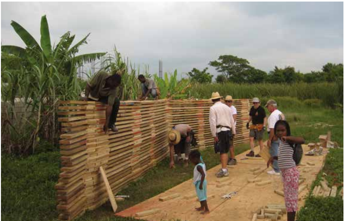
Members from the South Central States Mission Field help the Big Bridge Congregation in Jamaica put a roof on their new building.
